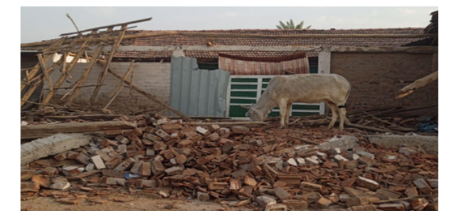
Figure 3: House demolished by bulldozers in Khamaria, Madhya Pradesh, April 2022. Source: Bebaak Collective, April 2022.
